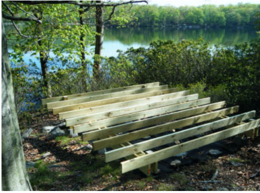
align joists
