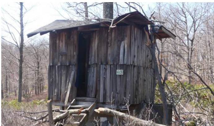
Winter storm damage photos by Derek Lomer
