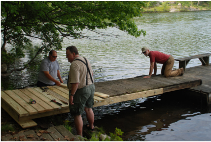
Guy, Ernie and Paul at work on the swim dock
