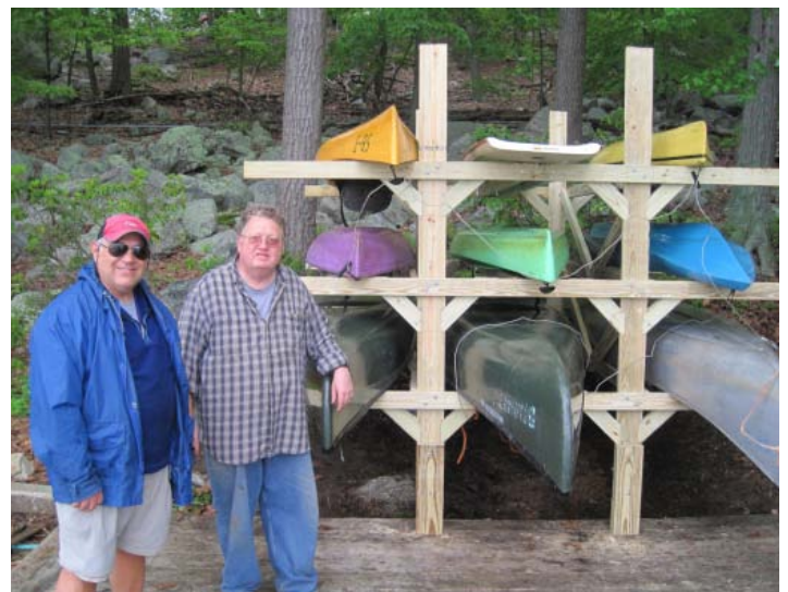
Many thanks to Paul Rondinone and Guy Lingley, seen here with their newly completed boat rack, which they built in two days. This is a major improvement to the camp! photo by Alex Wilkie
