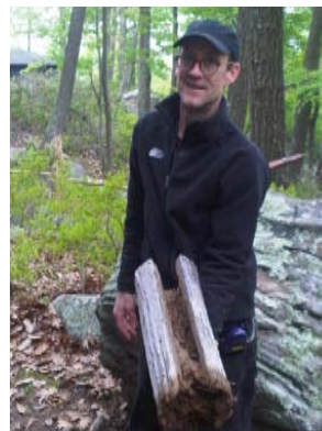
Termites ate the cores of the cabin 6 4 posts
